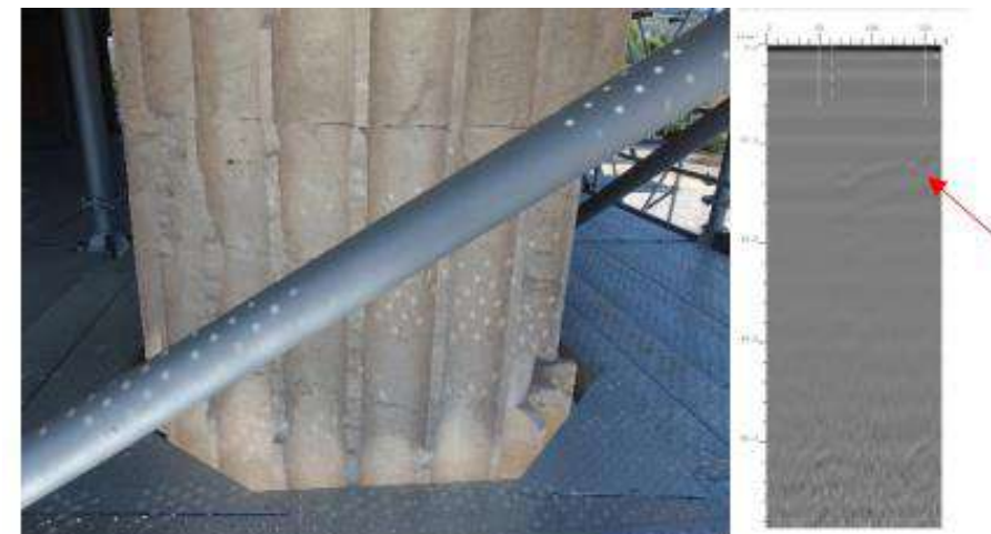
Column A1. Flut "α". No traces of lead between the drums
