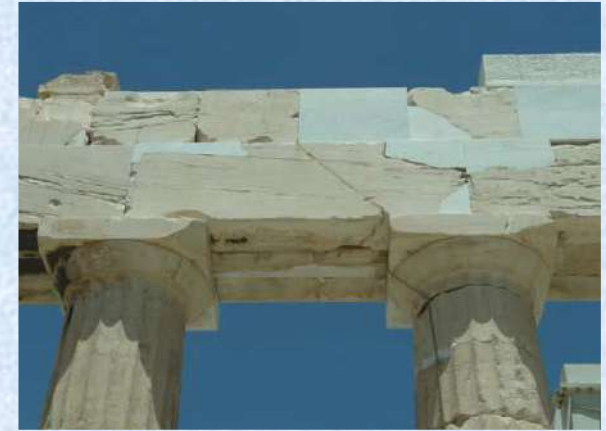
A restored epistyle of the Parthenon Temple on the Acropolis of Athens
